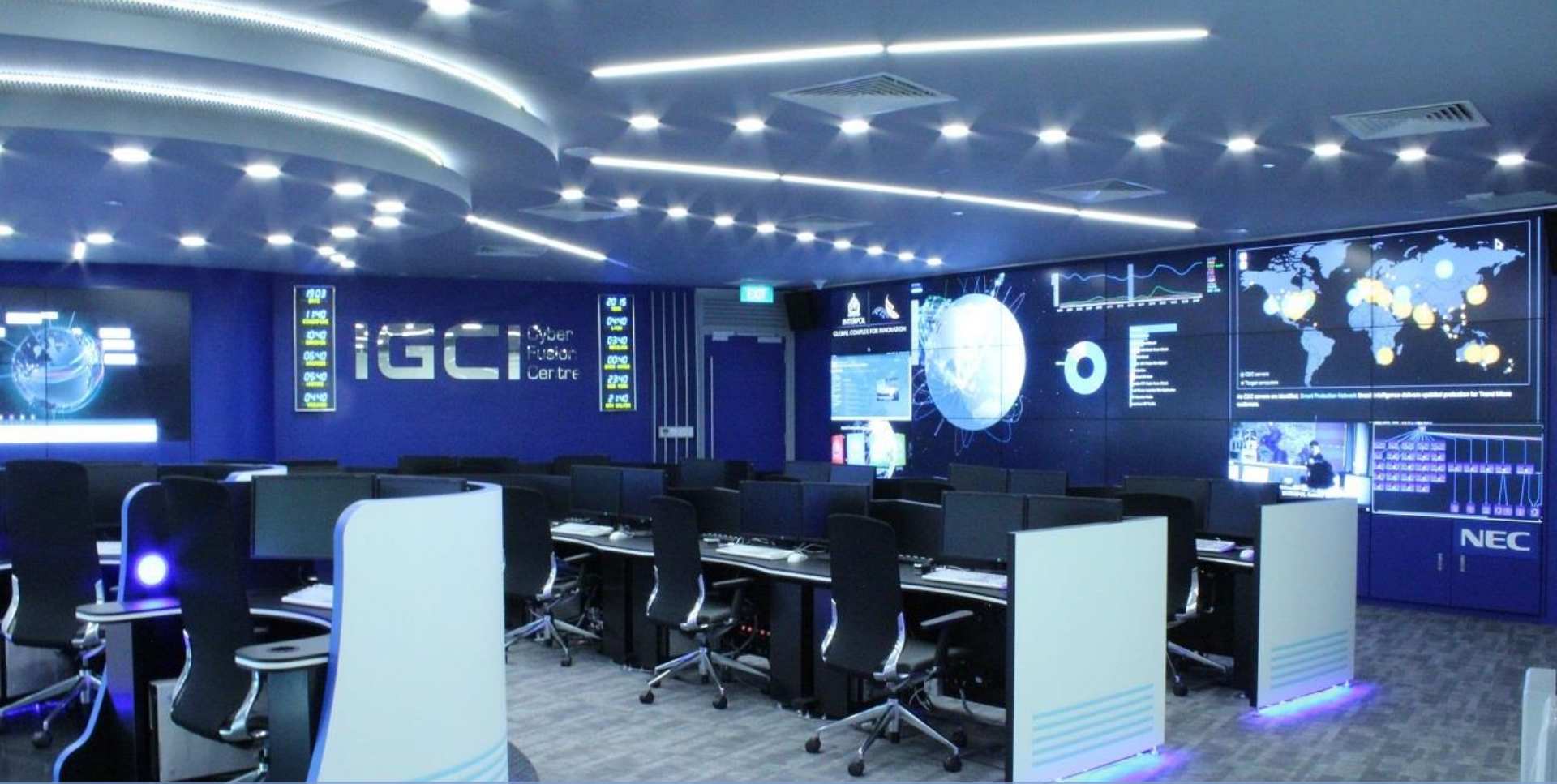
Cyber Fusion Centre (Main room)
